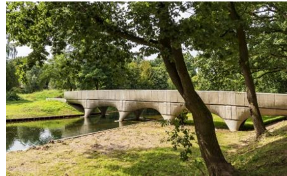
Fig. 5 The world's longest 3D printed bridge with a span of 29 meters [5].
