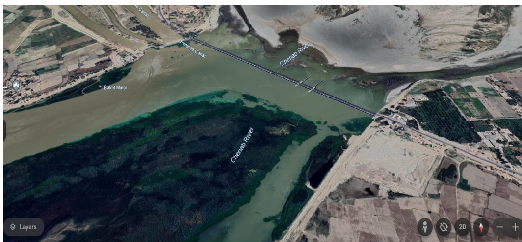
Figure 8. Aerial view of Panjnad barrage
