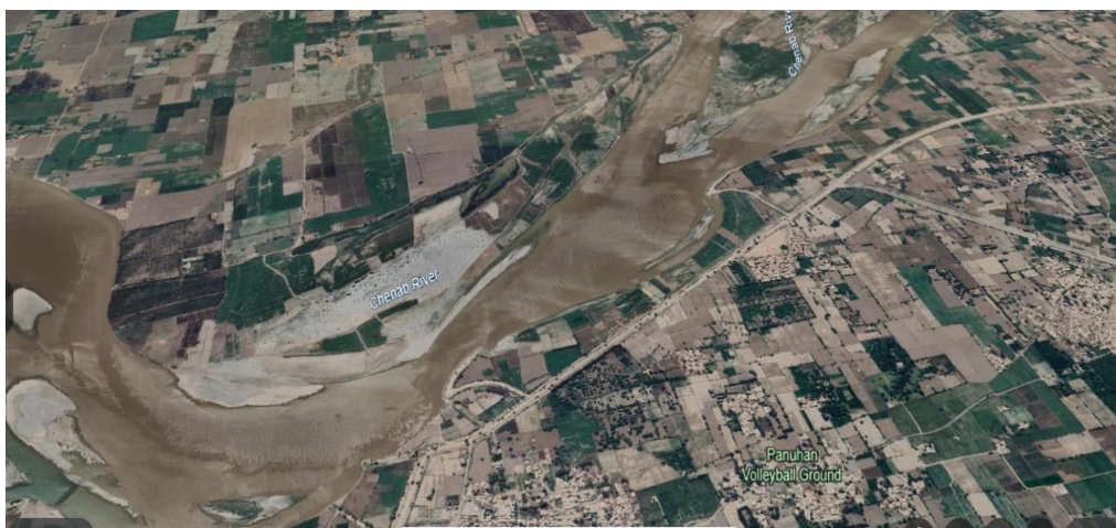
Figure 5. Vulnerable Reach RD30-52 RMB
