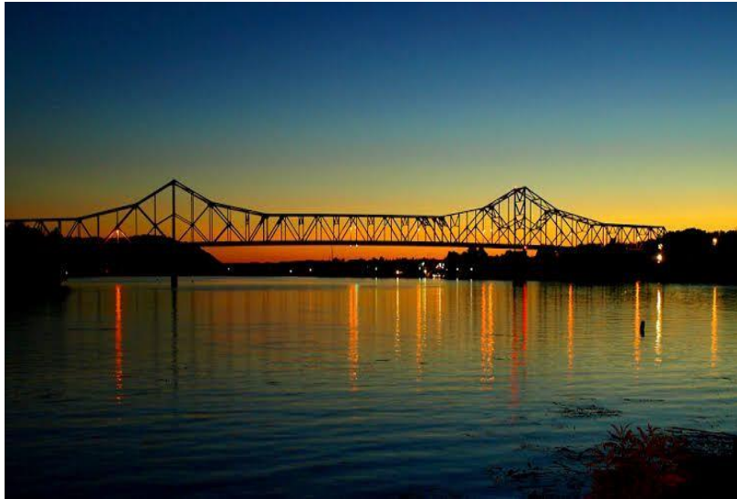
Fig. 5 Silver Memorial Bridge [16]
