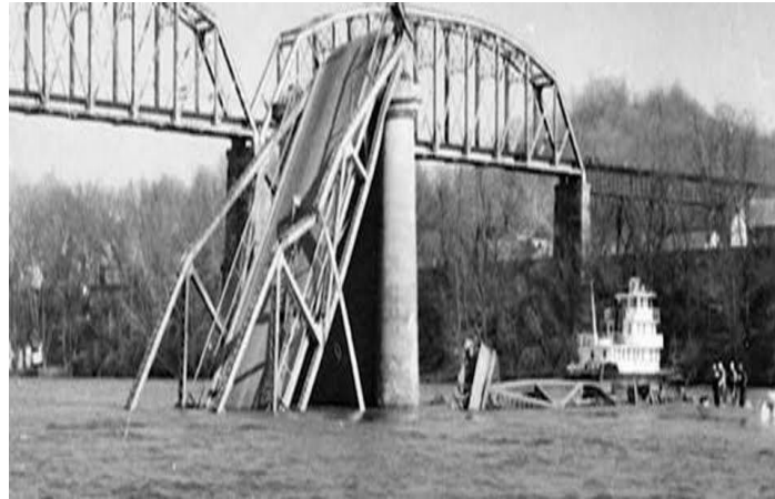
Fig. 4 Silver Bridge Collapse 1967 [17]
