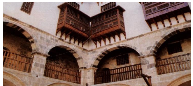
Fig. 9 Interior shot showing the facades after restoration
