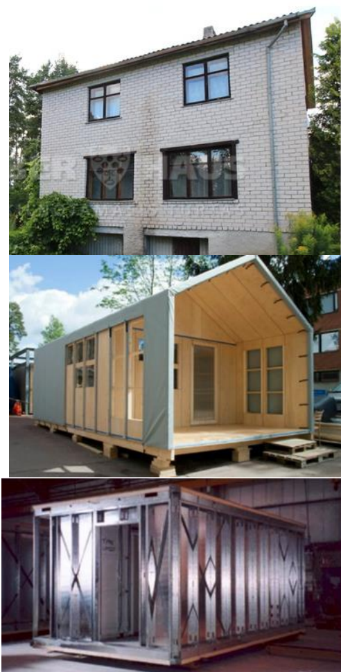
Fig. 4. A. Building with calcium silicate bricks [38]. B. Wooden-frame modular construction [39]. C. Metal-framed modular construction [40].
