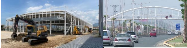
Fig. 8. A. Prefabricated metal building, Tirana, Albania [45]. B. Prefabricated metallic bridges, Tirana, Albania [46].
