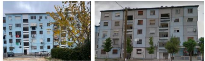
Fig. 5. Prefabricated residential buildings, Manhattan Street, Kamez, Tirana, Albania [44].
