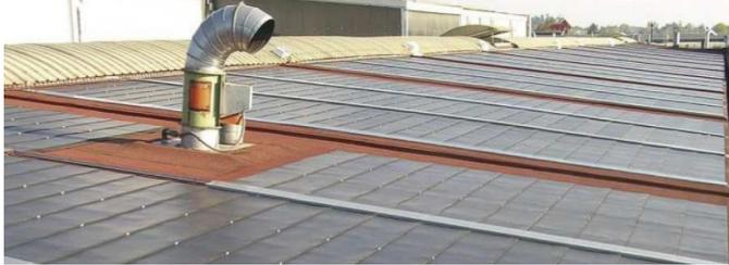
Fig. 5. Modular building equipped with PV system Tegola Solar [27].
